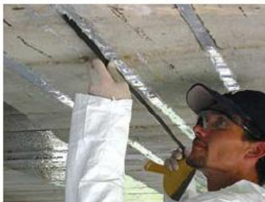
Inserting CFRP
