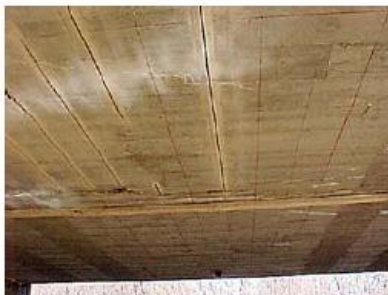
Groove is cut into element
