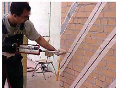
Filling groove with structural adhesive
