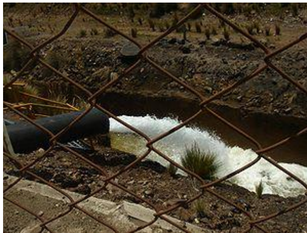
Fig. 1-1. Industrial wastewater effluent with neutralized pH from tailing runoff taken in Peru.
